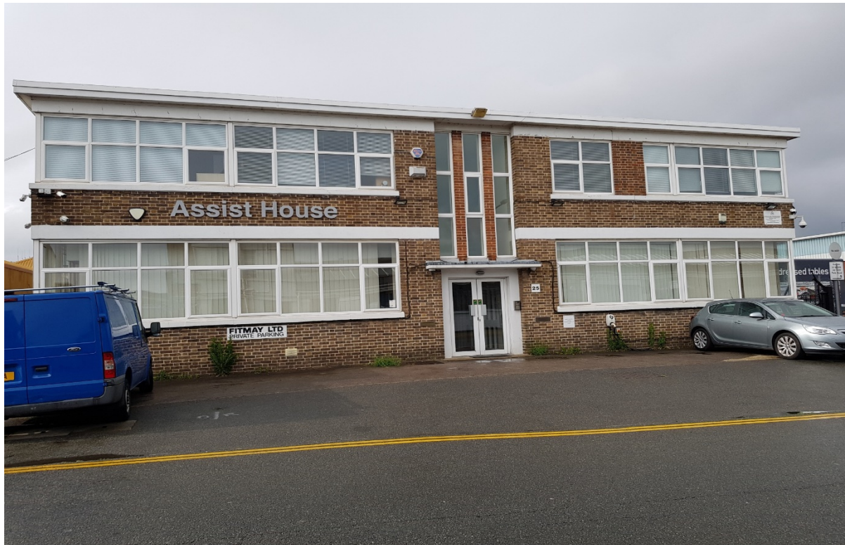
Assist House, 25 Lombard Road. (Fitmay House)
